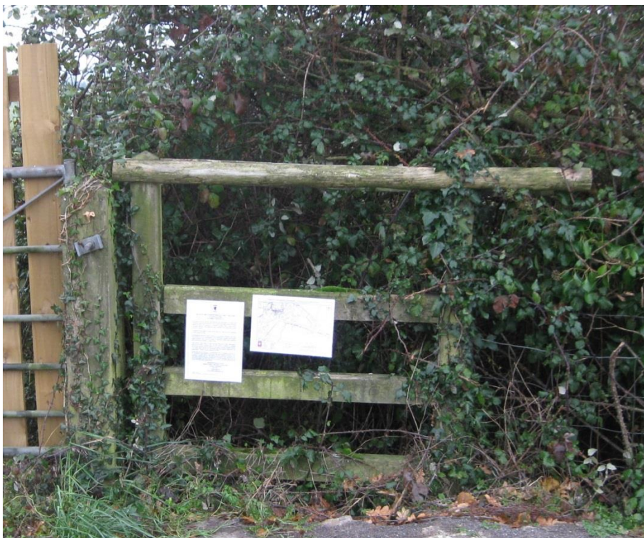
The wooden structure to the west of the field gate opposite Manor Farm at point B. The notices were placed by SCC as part of the consultation process relating to the investigation of this case.
